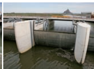
STAGE 3 The gradual opening of the gates underneath (underflow) allows for controlled releases of water to extend the effects of the ebb tide.
