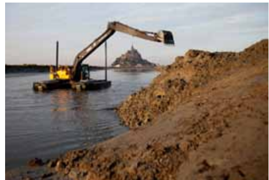
The «Big-Float» in the Couesnon estuary.
