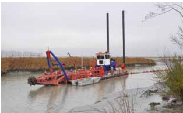
Suction dredge on the Couesnon
