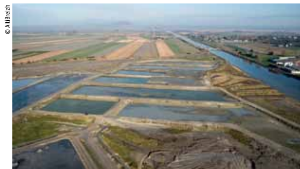
Silt decanting pots, northern section of the Moidrey cove – January 2013.
